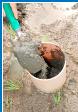
THE SOIL inside the tube is removed after sticking it into the ground.
